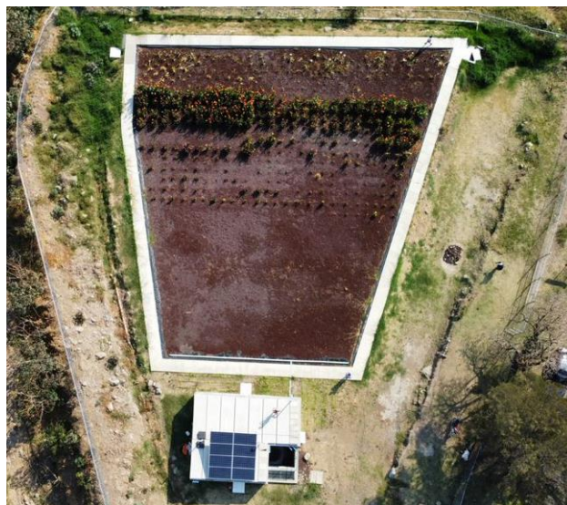
Figure 1. Aerial view of Atequizayán WWTP.
