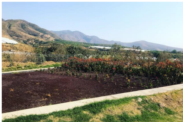
Figure 2. Lateral view of horizontal subsurface flow constructed wetland (HSSF).
